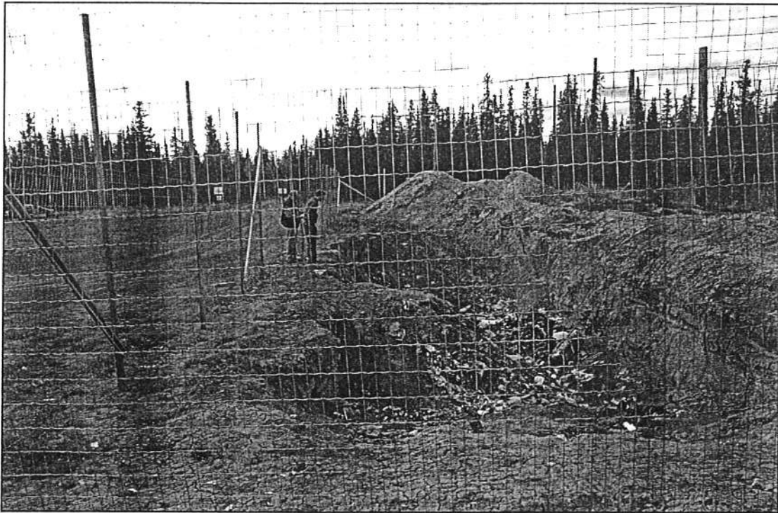
Photo 1. Canyon Creek Trench and Fencing
