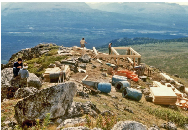
The Kusawa Tower under construction in 1983.
