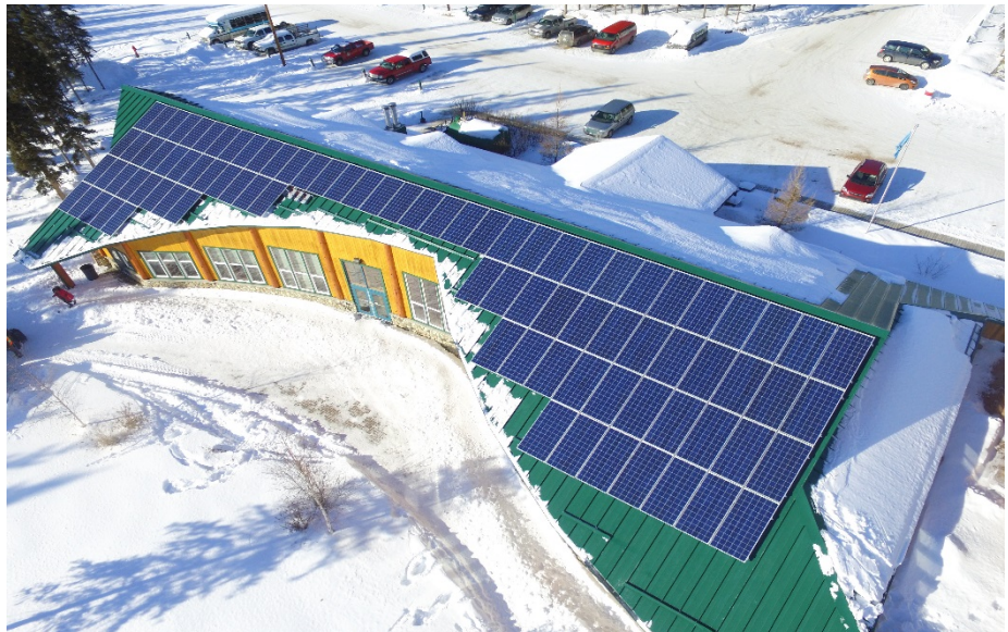
Solar array on Na-Cho Nyäk Dun First Nation's Government House in Mayo. Photo: Solvest.
