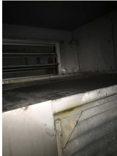
Figure 24: HRU-C1 Face-and-Bypass Dampers (from both sides)
