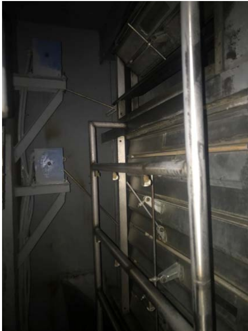
Figure 24: HRU-C1 Face-and-Bypass Dampers (from both sides)
