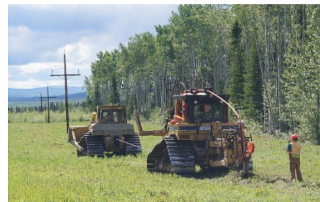
Conventional bury for areas with non-sensitive ground conditions. Generally involves two bulldozers cabled together.
