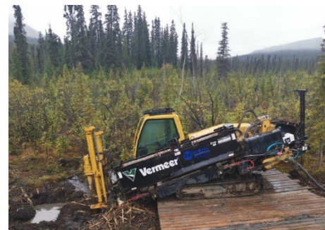
Horizontal directional drill and drill pad.
