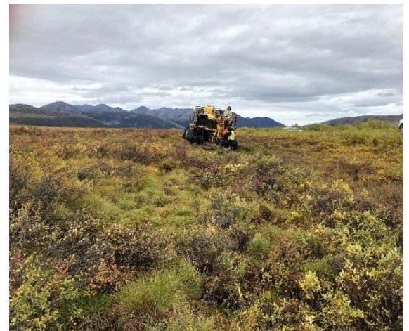
Final result of laying conduit with the Rolligon plow.
