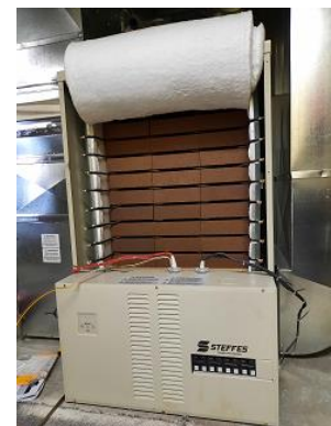
This brick-based ETS unit is an example of a system that stores electricity as heat.
