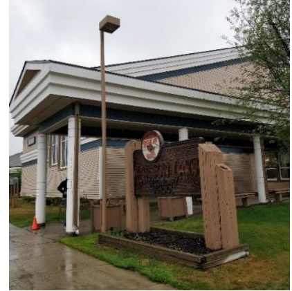
Watson Lake High School is heated with waste heat from the town's generators.
