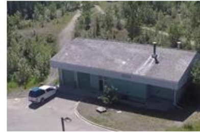
The biomass system is currently being installed in the boiler building at Elijah Smith Elementary School in Whitehorse, Yukon.
