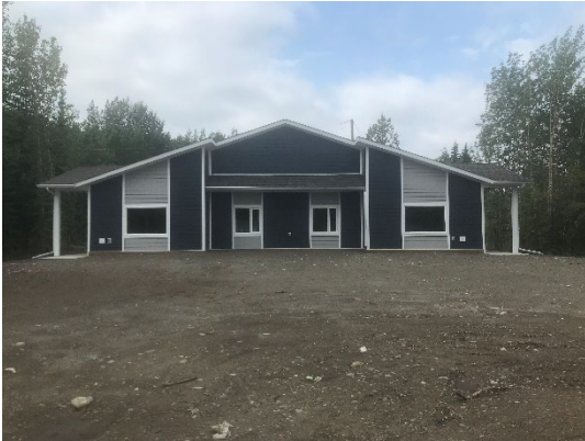
Carmacks duplex, purpose built to be comfortable and accessible homes.
